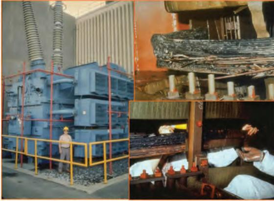
Figure 2-33. Damaged transformer at the Salem Nuclear Plant.
